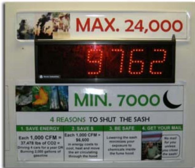
**Figure 6: Hood airflow display in one of Harvard's chemistry labs**
