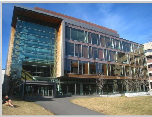
Northwest Labs Building Cambridge, MA 02138
